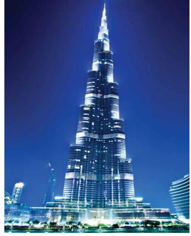
In April 2008, a new world record height of 606m for pumping concrete was set on the Burj Dubai (now Burj Khalifa) Tower in Dubai. Unimix is looking at the high pressure peristaltic or piston pump technology behind this level of performance and the contribution that it can make to the latest generation of high-rise building projects.
